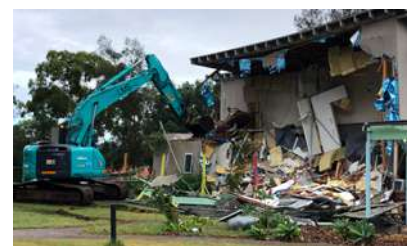
Demolition of the old cottages begins
